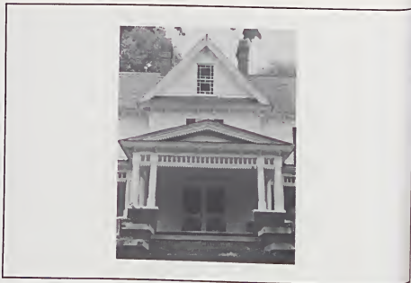
The beautiful raised porch of the R.L. Caviness House, Coleridge, showing bracketed frieze, pierced sawwork soffit and gable trim and bracketed cornice.
