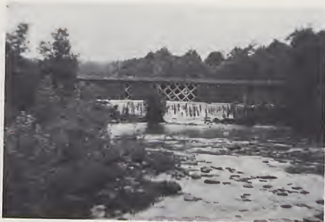
The Franklinville covered bridge ca. 1930.
