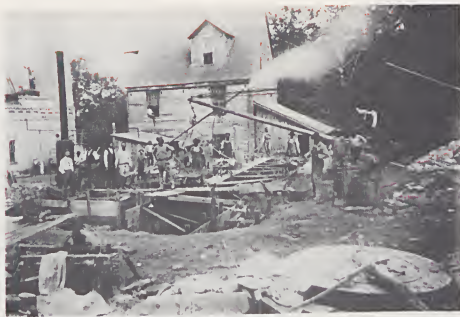
Franklinville grist mill (built ca. 1801) taken in 1912 when the foundations of the new roller mill were being built around it. The tiny old mill was destroyed soon after.
