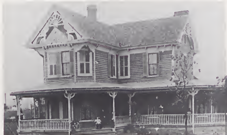
The first home built by industrialist Arthur Ross on the northeast corner of Sunset Avenue and Park Street was Asheboro's finest example of a decorative style which deserves to be called "Millwork Baroque." The end gable is a virtual catalog of some unknown company's millwork production. The house was subsequently moved and the present Colonial Revival style house was built on the site for Ross (courtesy Randolph Book 1779-1979 photograph collection in the Randolph Public Library).
