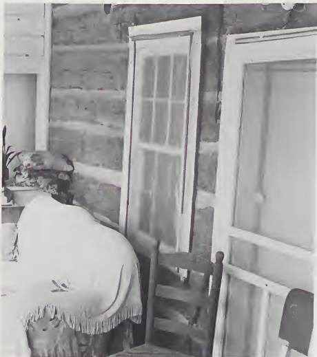
Contemporary photograph of the Enos Blair House porch, now a screened enclosure.
