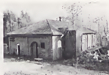
C:13 Power House
