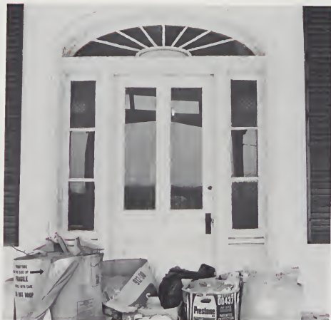
Paneled entrance to the Makepeace House, Franklinville, showing pulvinated frieze, sidelights and elliptical fanlight.
