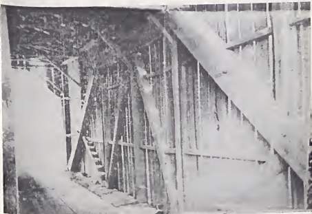
Documentary photograph showing the interior construction of the Skeen's Mill covered bridge, an example of mortise and tenon construction.
