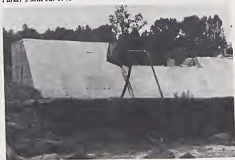
Asheboro's raw water reservoir dam.
