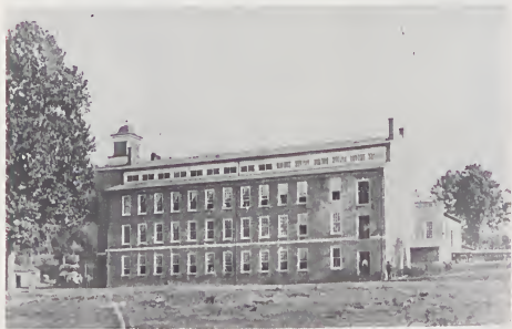
The 1846 Cedar Falls factory ca. 1900, viewed from the southeast. The monitor roof and chimneys are clearly visible. The stail tower and cupola at the west end are later 19th century additions (courtesy Randolph Book 1779-1979 photograph collection in the Randolph Public Library).
