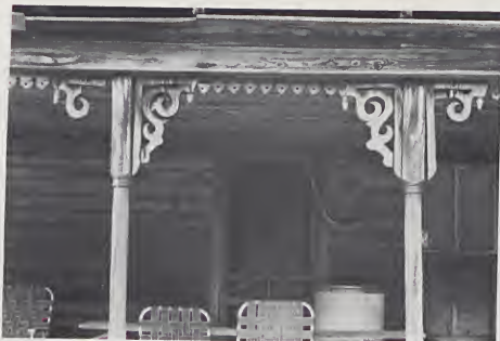
Detail of house in Coleridge Township showing sawnwork brackets, turned porch posts and pierced sawnwork soffit decoration.
