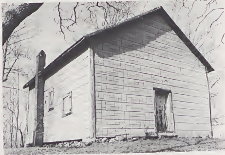
Sandy Creek Baptist Church, Liberty Township. Built in 1826, it is the oldest organized church and oldest surviving religious structure in Randolph County. Founded in 1755 by Separate Baptist Minister Shubal Stearns (courtesy Randolph Book 1779-1979 photograph collection in the Randolph Public Library).
