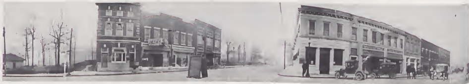
This panoramic view of the Sunset Avenue-Fayetteville Street intersection was taken ca. 1925 from the opposite corner of the ca.-1900 panorama. The Bank of Randolph, Capital Theatre and First National Bank are the landmarks of this important corner; all have been destroyed (courtesy Randolph Book 1779-1979 photograph collection in the Randolph Public Library).
