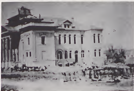
Two views of the present Randolph County Courthouse under construction in 1909 (courtesy Randolph Book 1779-1979 photograph collection in the Randolph Public Library).
