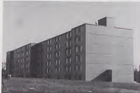
B-47 The Asheboro Summit housing complex located to the east, directly behind the former Fayetteville Street School.
