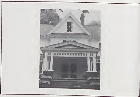
The beautiful raised porch of the R.L. Caviness House, Coleridge, showing bracketed frieze, pierced sawnwork soffit and gable trim and bracketed cornice.
