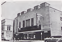
B:35 Cranford Building ca. 1932.
