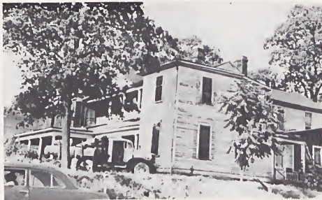
(C) View from the southwest as demolition begins.
