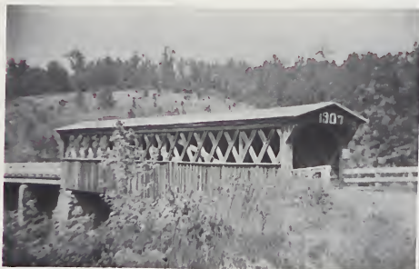
Fuller's Mill covered bridge, built in 1907.
