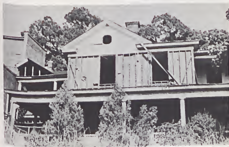
(D) The northwest wing under demolition.
