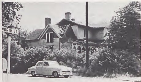
(B) Demolition begins in the summer . . .
