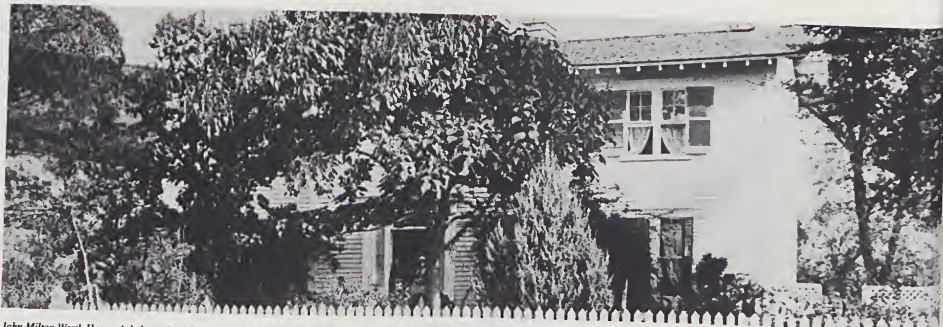
John Milton Worth House, Asheboro, in a documentary photograph taken ca. 1870. The original Greek Revival facade is visible here before the addition of an elaborate Eastlake-style porch ca. 1880.
