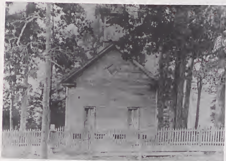
D:2 Methodist Episcopal Church ca. 1890 (Original photograph by H. M. Robins).
