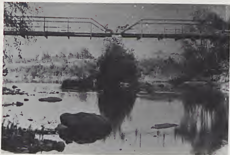
Central spans of the Island Ford iron bridge.
