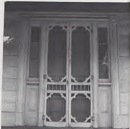
Entrance to the Lambert-Parks House, Franklinville, with Greek Revival style symmetrically-molded panels and corner blocks (Ruth Little).
