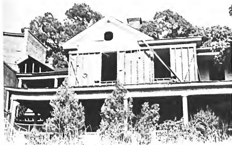
(D) The northwest wing under demolition.
