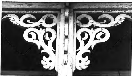
Elaborate sawn brackets of the Gregson-Pickard House, Randleman (courtesy Randolph Book 1779-1979 photograph collection in the Randolph Public Library).
