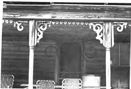
Detail of house in Coleridge Township showing sawnwork brackets, turned porch posts and pierced sawnwork soffit decoration.
