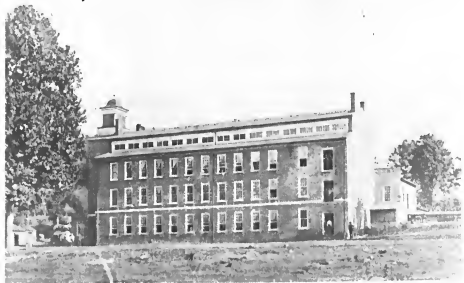
The 1846 Cedar Falls factory ca. 1900, viewed from the southeast. The monitor roof and chimneys are clearly visible. The stair tower and cupola at the west end are later 19th century additions (courtesy Randolph Book 1779-1979 photograph collection in the Randolph Public Library).
