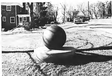
This pair of iron balls and granite troughs were used to grind gold at the Gray mine near Asheboro. Made in Belgium, they were shipped to Wilmington in the 1840s, were barged up the Cape Fear River to Fayetteville and were brought to Randolph County by wagon. Presently located on Marmaduke Circle, behind the home of J. D. Ross, Jr.
