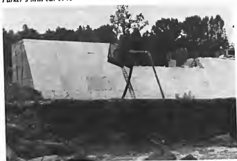
Asheboro's raw water reservoir dam.
