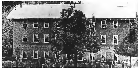
Western side of the Franklinville Manufacturing Company factory, as it appeared in 1874. A cupola is faintly visible at the north end of the roof. The demarcation line between the original 1838 first floor masonry and the darker post-1851 masonry is evident.
