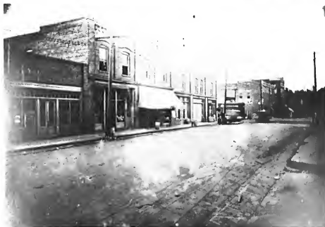
B:23 The Stedman Block looking east on Sunset Ave. ca. 1923.
