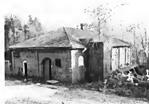
C:13 Power House
