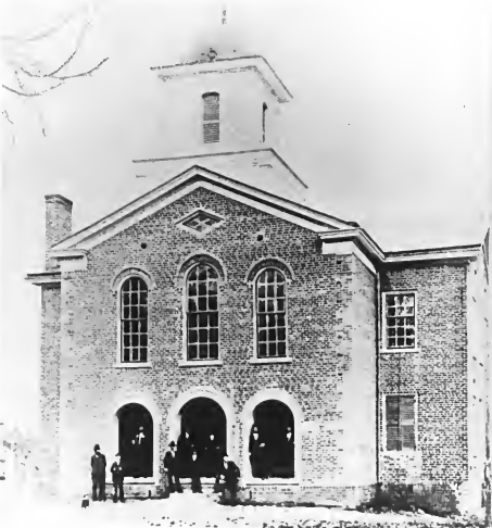
This photograph of the Randolph County Courthouse was probably made ca. 1890. The original two-story 1839 courthouse is visible behind the entrance pavilion added in 1876. This is the south facade of the building (courtesy Randolph Book 1779-1979 photograph collection in the Randolph Public Library).
