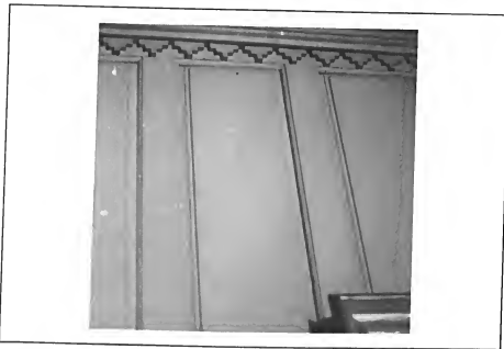
Interior photograph of the Coletrane House, New Market Township, showing the embattled molding crowning the paneled chimney piece.
