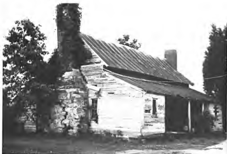
Frazier double-pen log House, New Market Township; built ca. 1780; demolished 1981.
