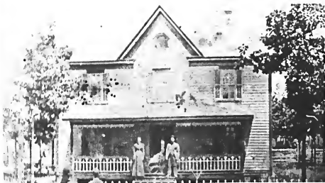
The Clark Cox House was located near the roller mill. The form of the center-hall plan central gable house is not unusual but the porch and wooden fence are attractive exhibitions of the house carpenter's facility in combining millwork products for decorative effect.
