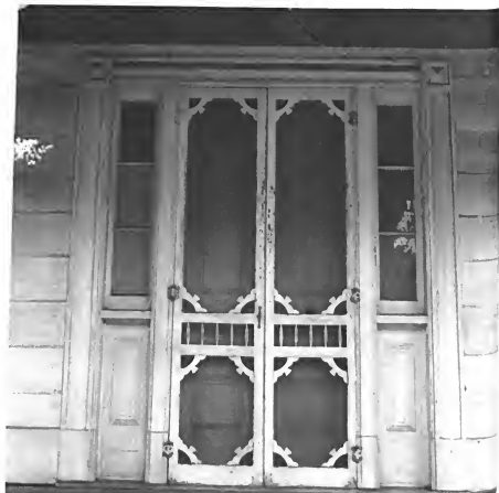
Entrance to the Lambert-Parks House, Franklinville, with Greek Revival style symmetrically-molded corner blocks (Ruth Little).
