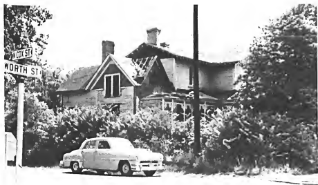
(B) Demolition begins in the summer . . .
