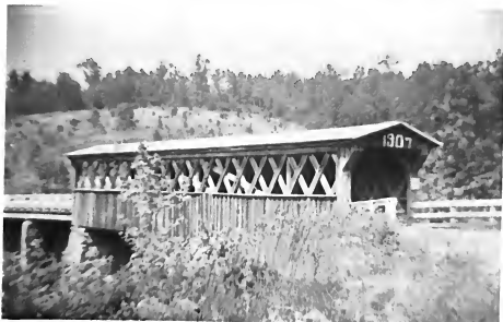
Fuller's Mill covered bridge, built in 1907.
