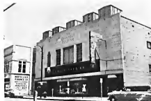
B:35 Cranford Building ca. 1936.
