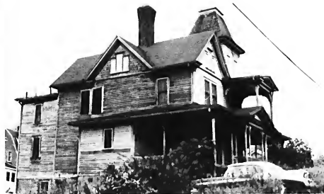
Roller mill executive W. J. Scarborough built this large house in the late 1890s. Its mansard-roofed tower was one of the county's few examples of the "Second Empire" style.
