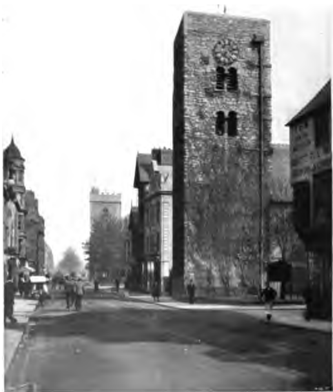
PRE-NORMAN TOWER (ST. MICHAEL'S, OXFORD)
