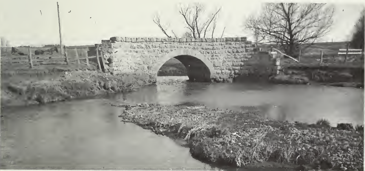
The Old Stone Bridge, an early landmark near Lanark.
